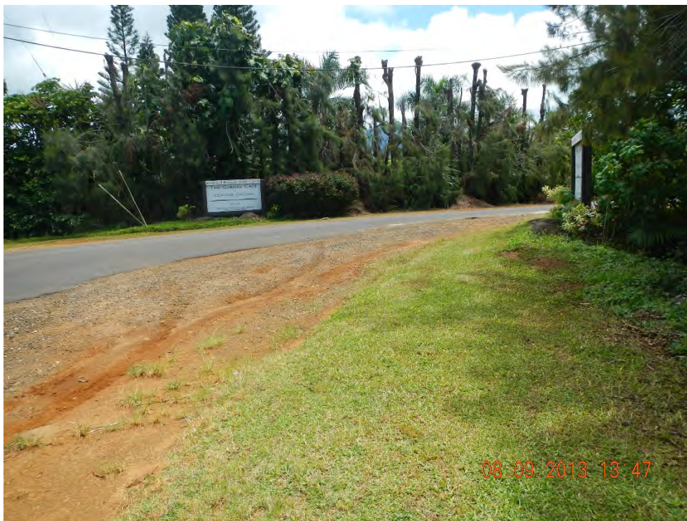
Photo 2: The paving along the road/entrance to Kuawa Road clearly needs to be widened to accommodate vehicles as evidenced from ruts and tire tracks in the dirt.
