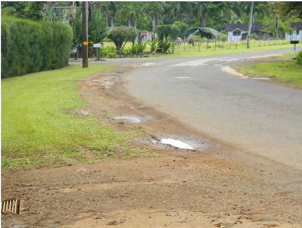
Photo 10: Potholes on the left just past our properties driveway toward the Manager's House Driveway; standing water remains in the ruts and potholes from the night before. Notice the numerous patches on the road itself directly in front of the Manager's House Driveway.
