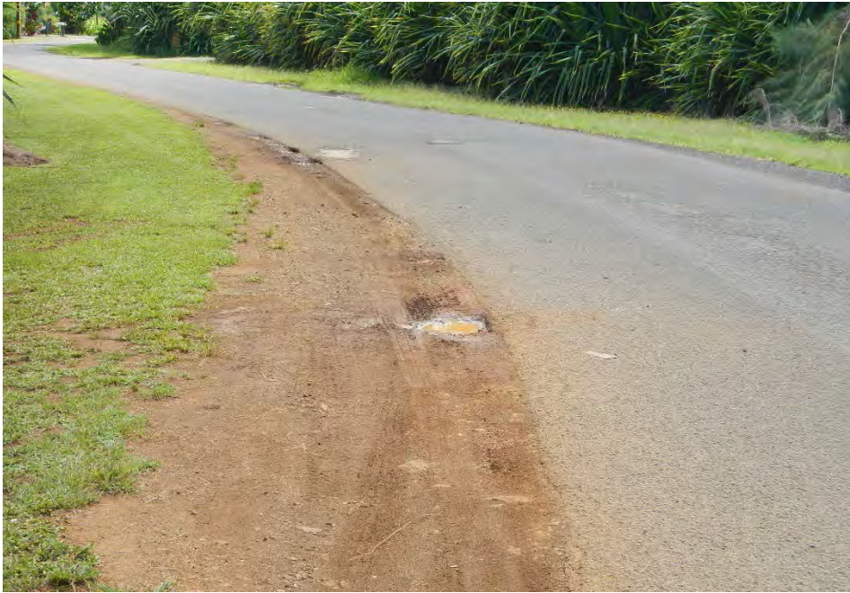
Photo 7: Potholes along the margin of the road.
